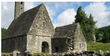
St Kevin's Church at Glendalough, Wicklow
